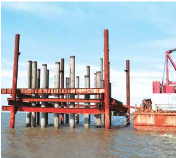
Construction of Tan Thuan wind turbines foundation
