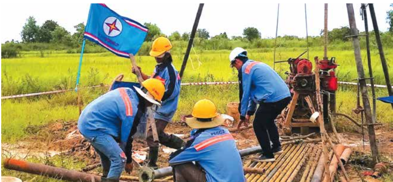
Geological Investigation of Phnom Penh airport - Phase 2
