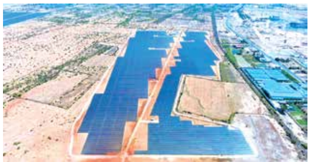
Phuoc Ninh Solar Power Plant (50MWp)
