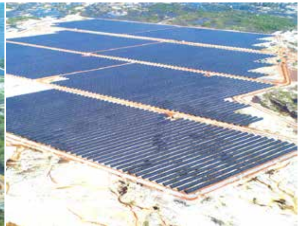
Gio Thanh 2 Solar Power Plant (50MWp) - EPC
