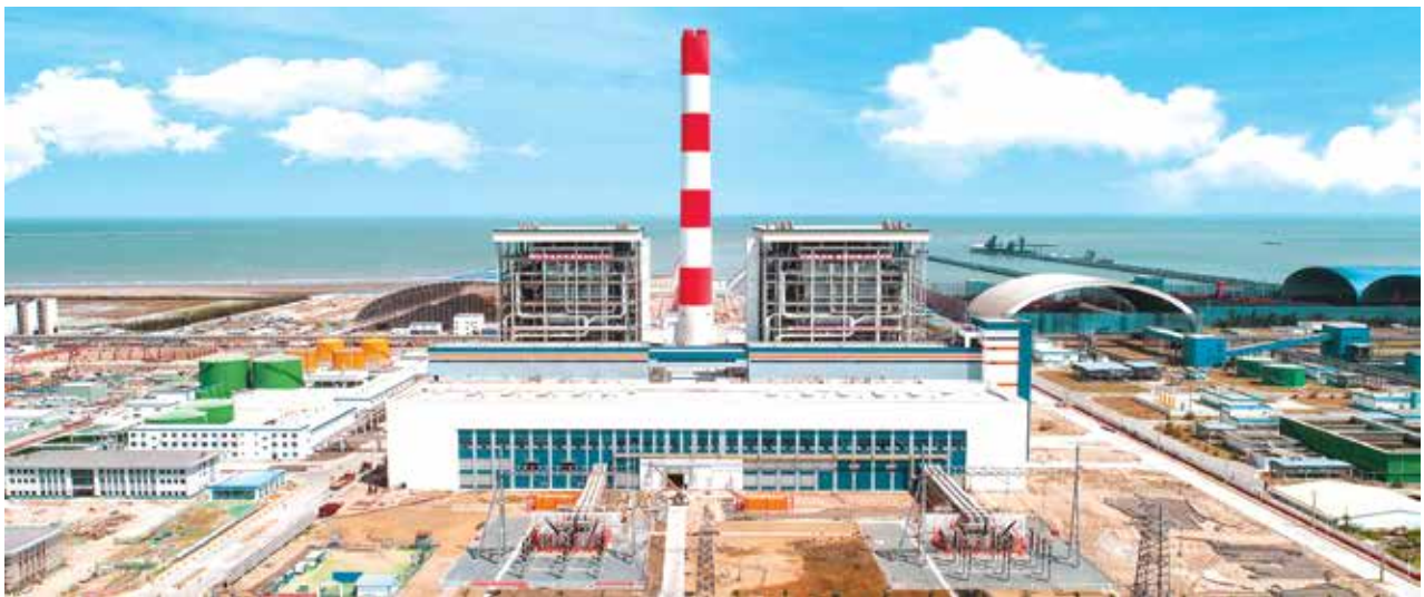
Duyen Hai 2 Extension Thermal Power Plant
