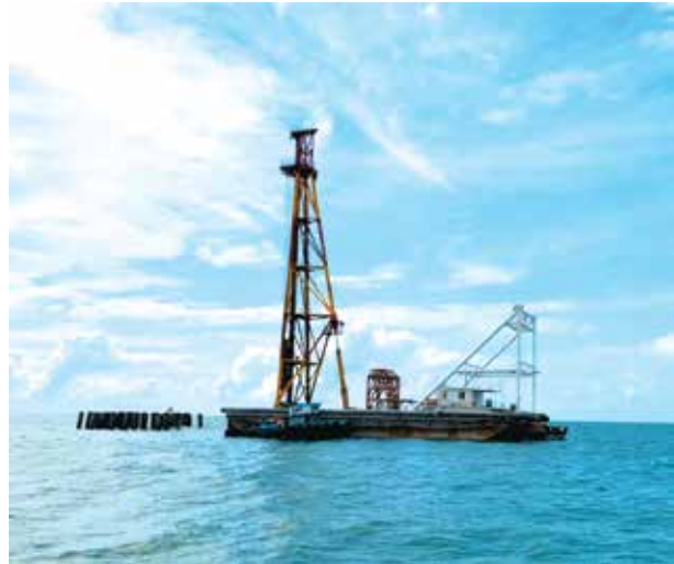
Construction of 220kV Kien Binh - Phu Quoc transmission line
